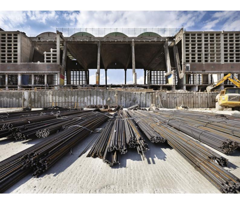
The foundation plate for the double office tower is about three metres thick. Approximately 4,200 tonnes of steel were required to reinforce the concrete.
