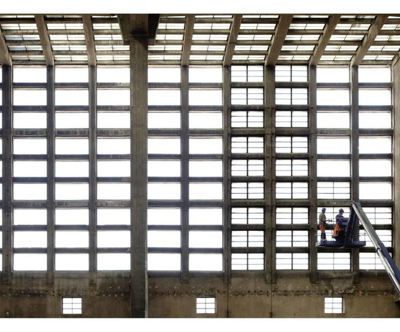
Interior view of the Grossmarkthalle's concrete grid facade. The restoration of the Grossmarkthalle is an important aspect of the construction works. The fundamental appearance of the building will be retained, with its facades and surfaces being restored in line with the preservation order.
